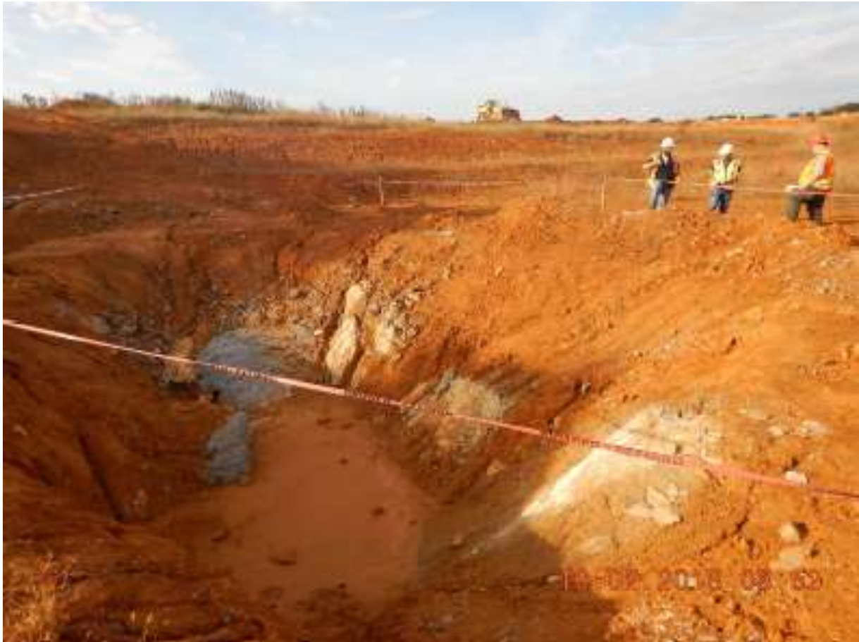
Sinkhole in Rockwool's Basin #1 – October, 2018
