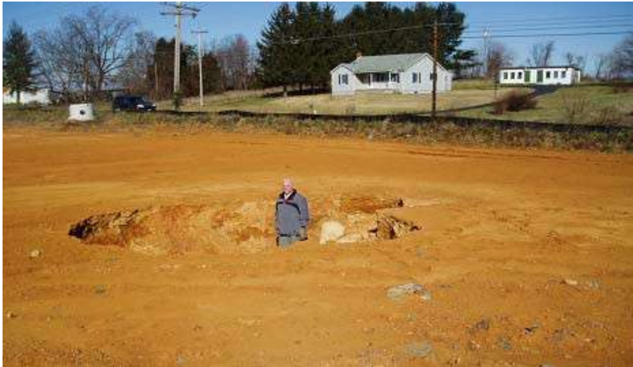
(Sinkhole at the abandoned Tackley Mills subdivision at the intersection of Old 9 and Wiltshire Bld. The sinkhole grew large enough to threaten Old 9)
