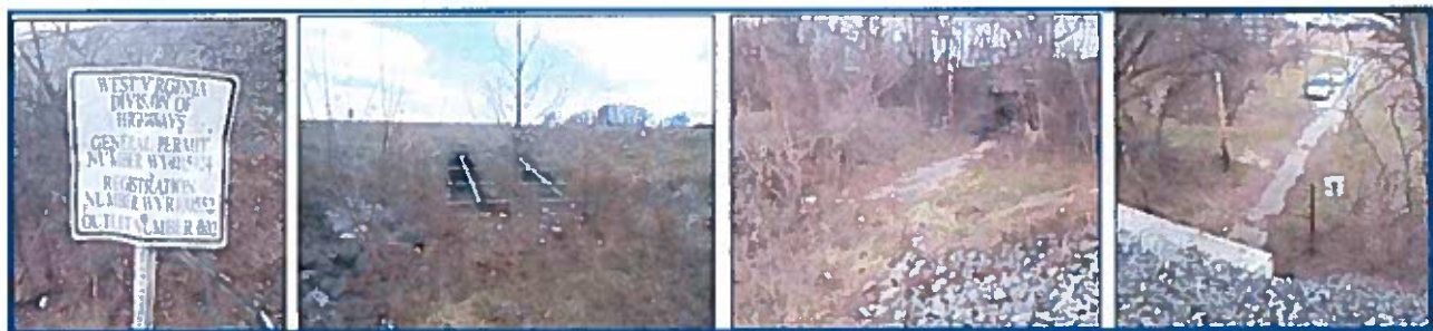
Figure 6 – CSX Rail Tunnel Drainage
