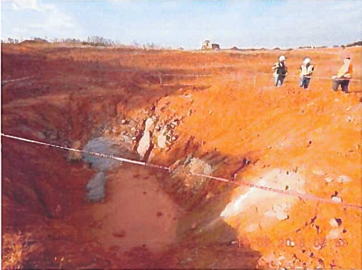
Sinkhole in Rockwool's Basin #1 – October, 2018
