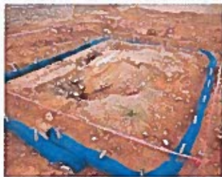
Close-up view of potential sinkhole located in the reuse pond with protection.
