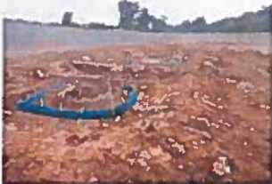
Problems with earth berm and blue tarp protection identified in the reuse pond.
