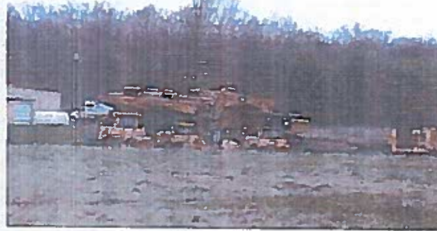
Trucks with heavy equipment at the Rockwool site in Ranson, W. Va. The site is located on a cleared 136-acre plot near W.Va. 9.
