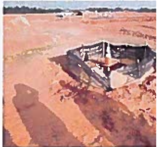
Sinkhole # 7 capped with concrete deep inlet structure.
