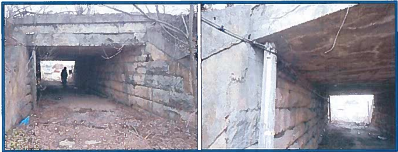
Figure 5 – CSX Rail Tunnel
