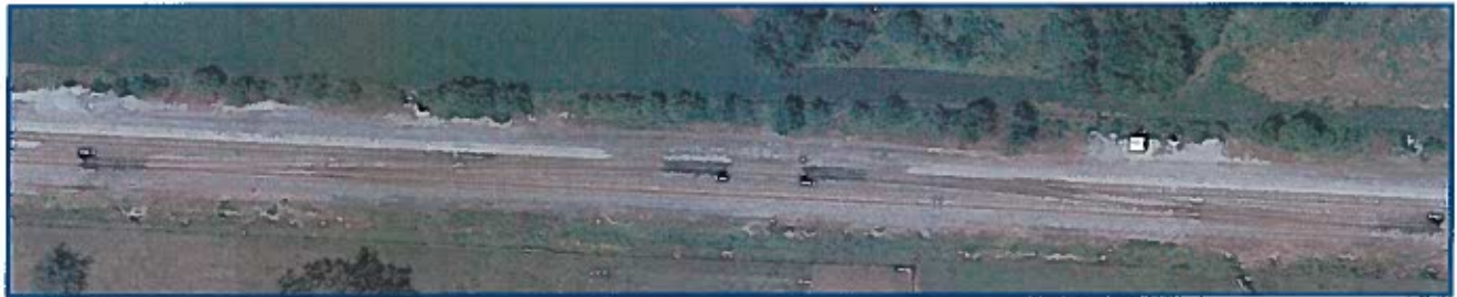
Figure 10 – CSX Track Interlocking Southeast of Jefferson Orchards
