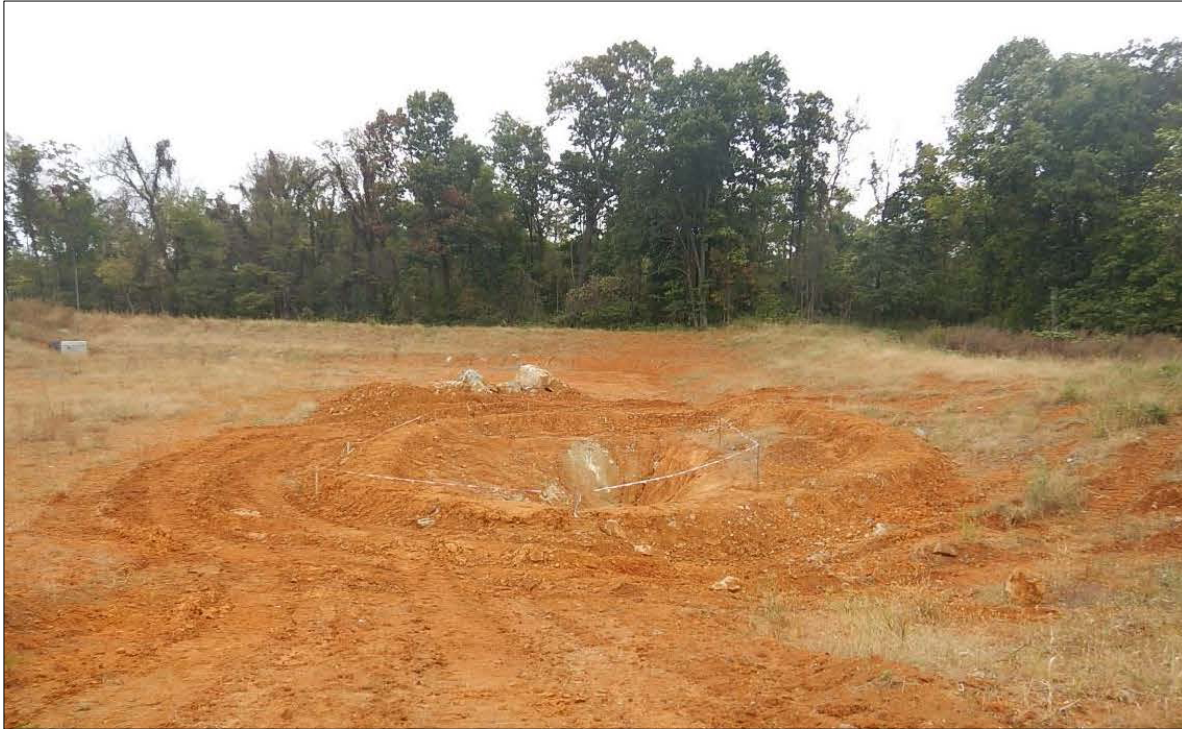
Figure 10. Sinkhole in Sediment Basin #1 (WVDEP 2018d) (photographer not named).
