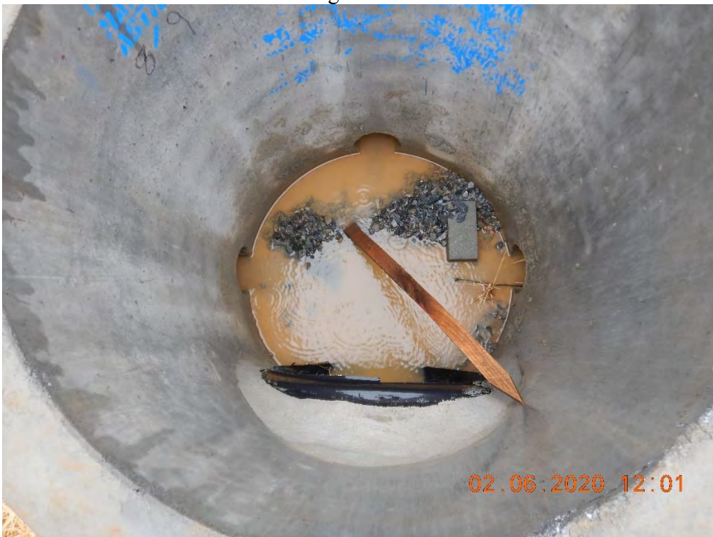
Sediment laden water leaving Sediment Basin through orifice in riser.
