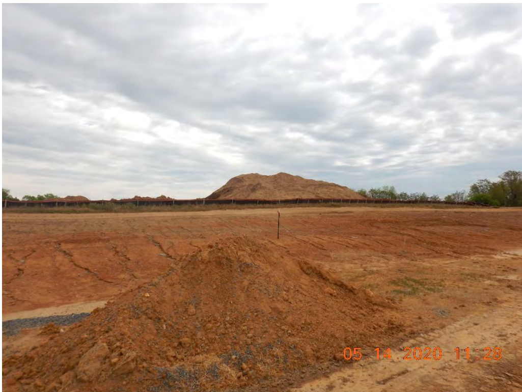
Stockpile area has not germinated within 30 days after seeding.
