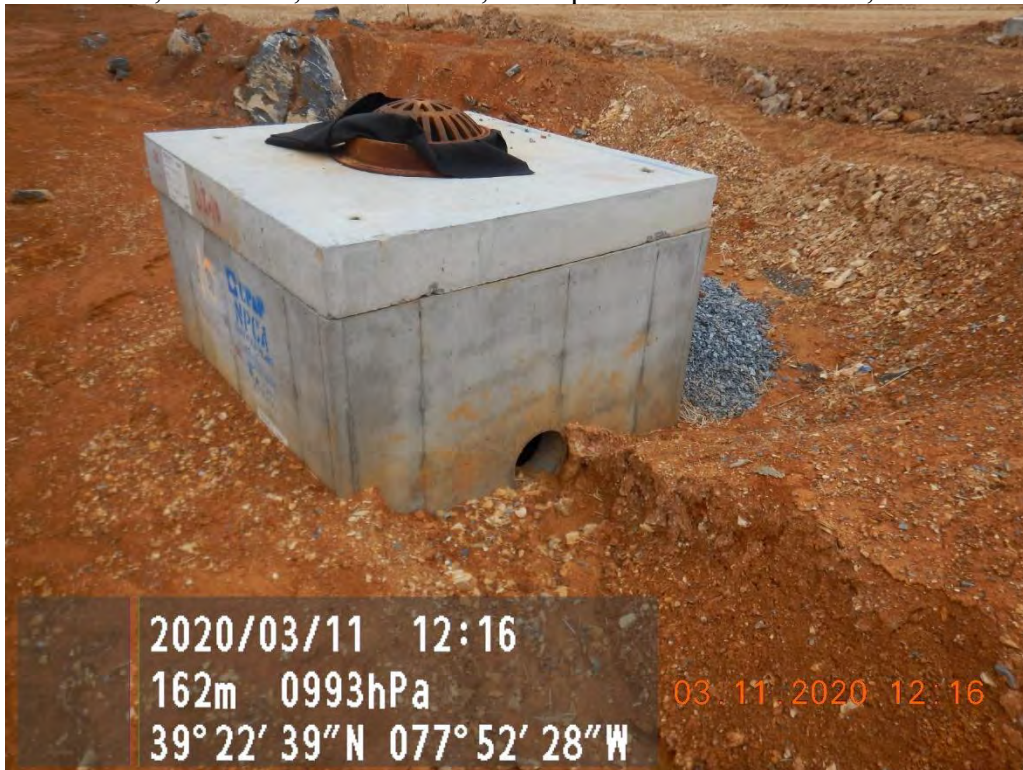
Drop inlet with out protection on side after maintenance was performed. Was immediately corrected upon notification.
