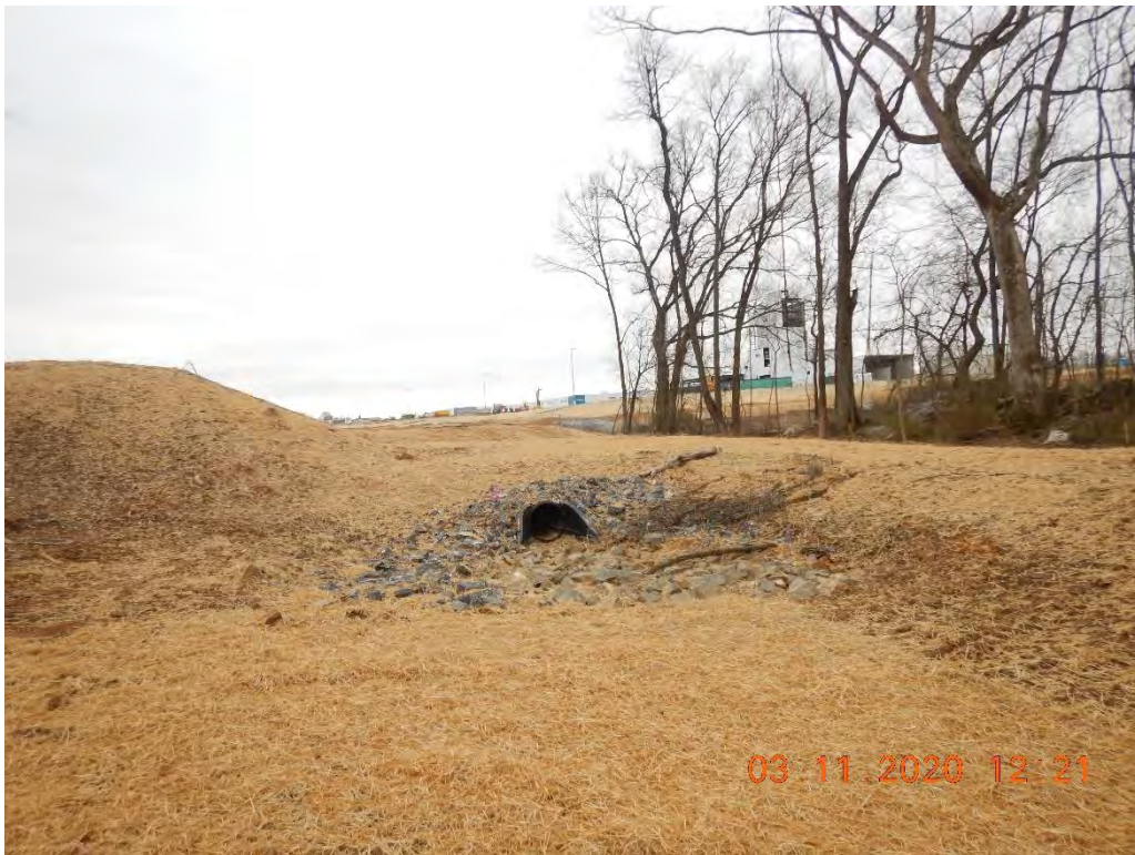
Outlet marker was not place at outfall of basin 1 yet. They are being made and will be posted within the next 24 hrs.
