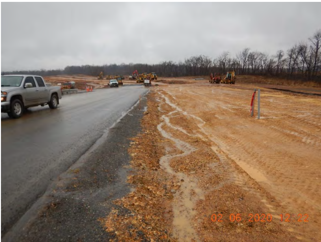
Diversion along Northport Ave. does not have rock check dams as indicated on plan sheet 9.
