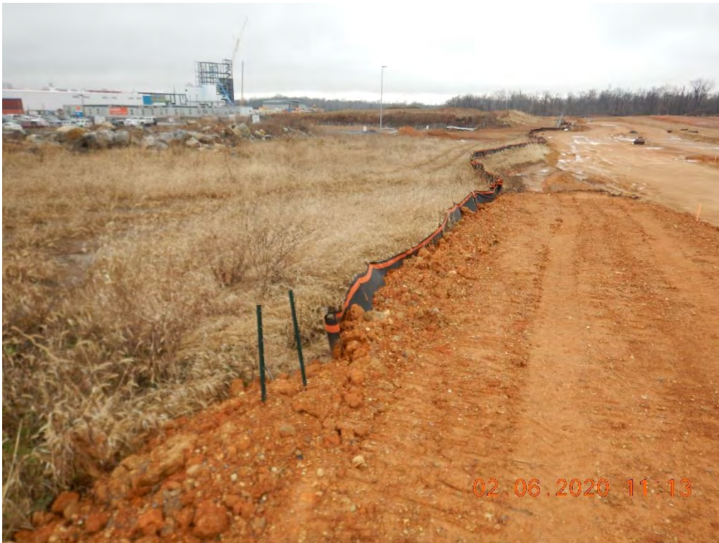
Where soil is being pushed up against silt fence, there is no holding capacity to allow proper filtration before being overtopped.
