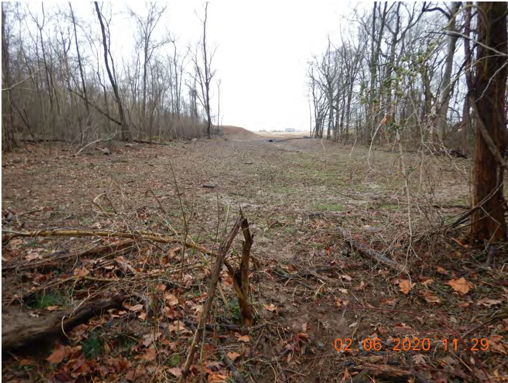
Diversion channel #1 and rip rap apron #2 not installed at time of inspection.
