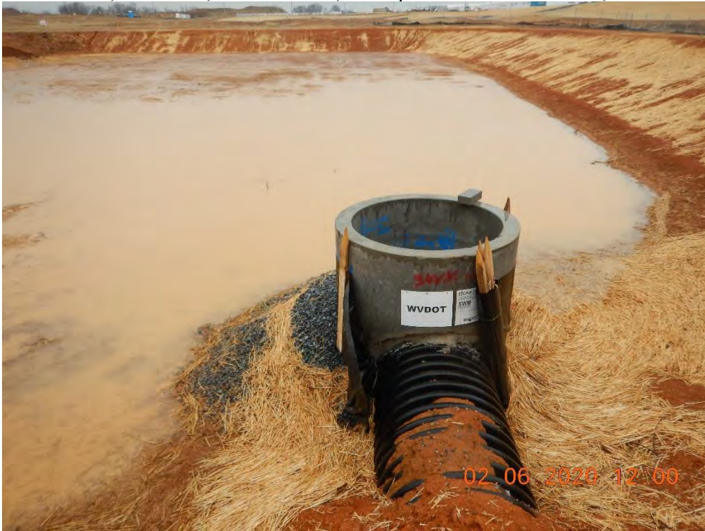
Sediment basin is not being operated correctly and is allowing sediment laden water to leave the site without going through an appropriate erosion control device. Sediment basin should be set up to 50% percent wet/dry compacity. At time of inspection it is set up for stormwater retention with the orifices at bottom grade of basin.
