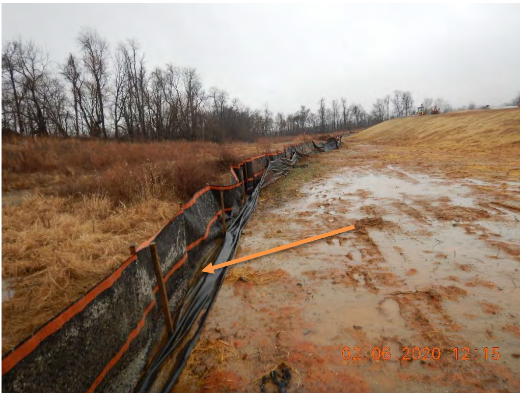
By-pass under silt fence that allows sediment laden water to leave the site.
