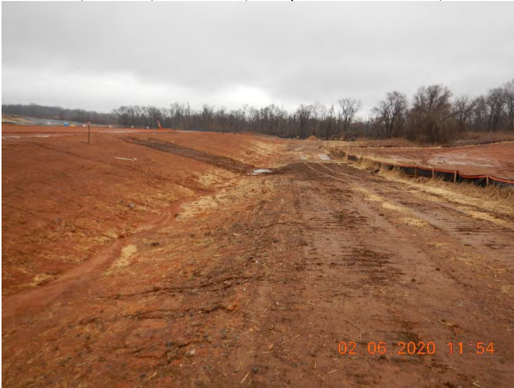
Diversion channel not installed per plan sheet details with ECM and rock check dams.
