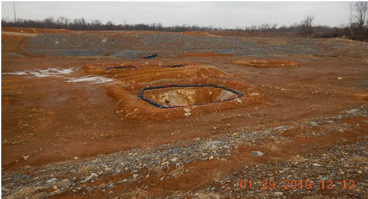
Figure 9. Several sinkholes in the Reuse Pond (WVDEP 2019a) with temporary structures to minimize the transport of sediment into the karst aquifer (photographer not named).
