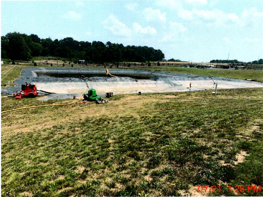
Forebay pond discharges to outlet 001
