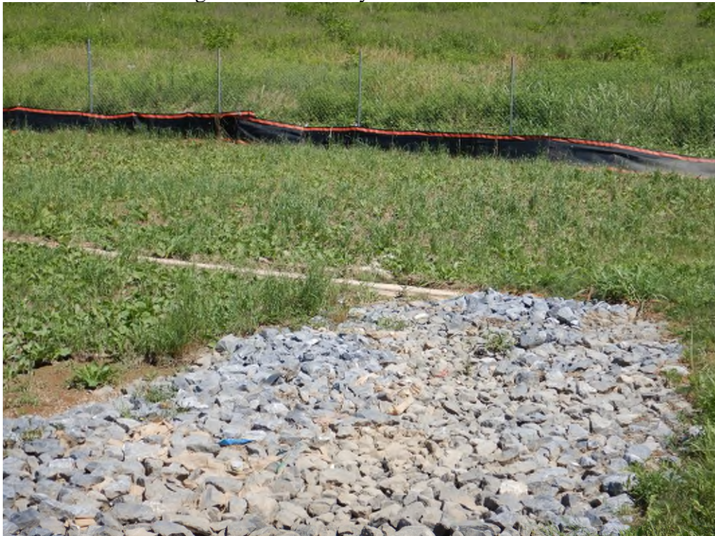
Level Spreader installed per SWPPP.
