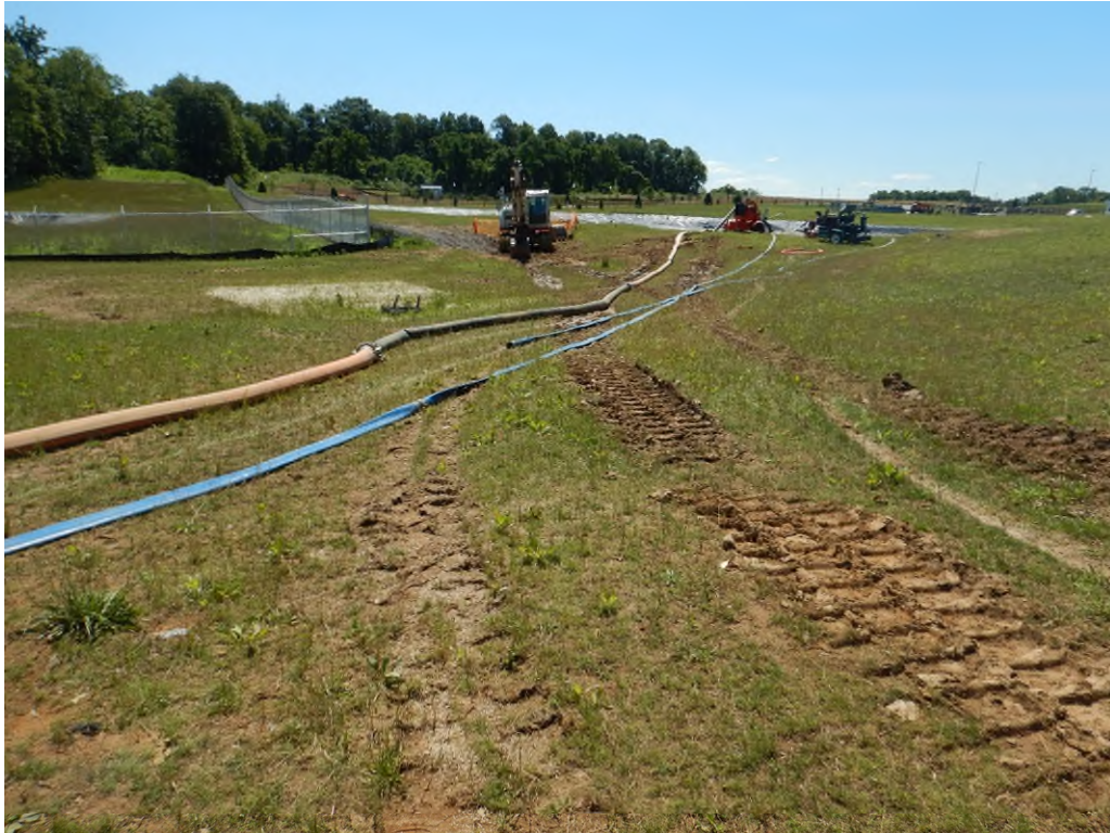
Work being done on Butterfly Valve for Stormwater Pond
